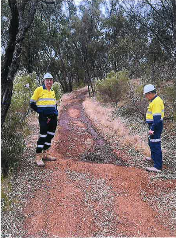
Photo 11: Resources Regulator undertaking a safety inspection of the OCE. Observing a water leak from the PSC reservoirs. Photo taken 1 December 2025.
