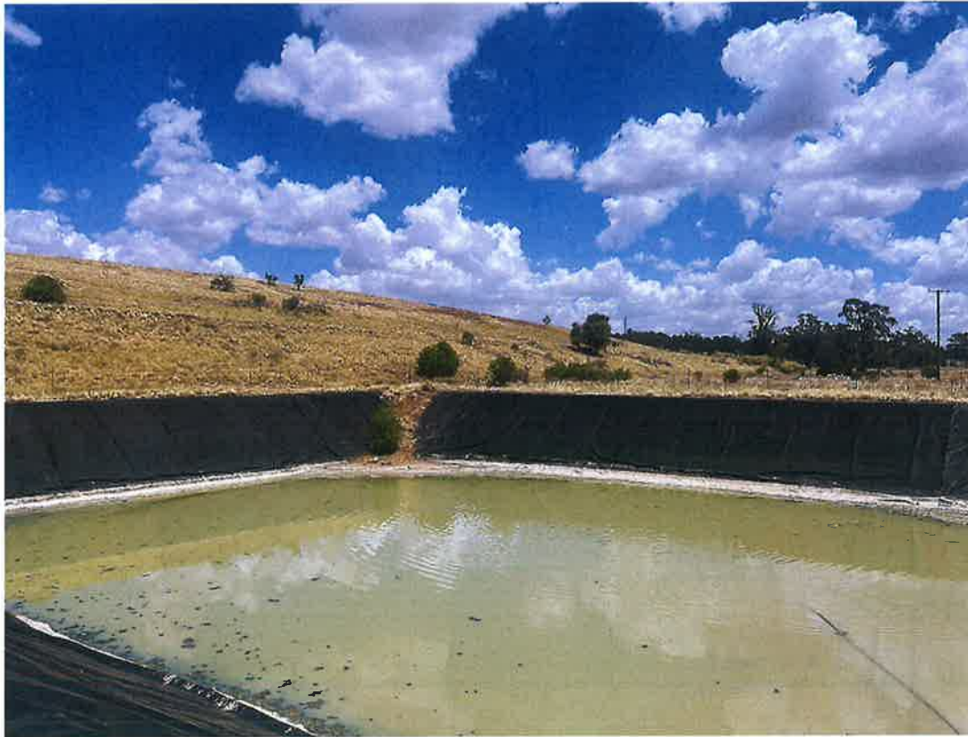
Photo 3: Pregnant overflow pond status 4 February 2025. Wildlife egress ramp mid-image.
