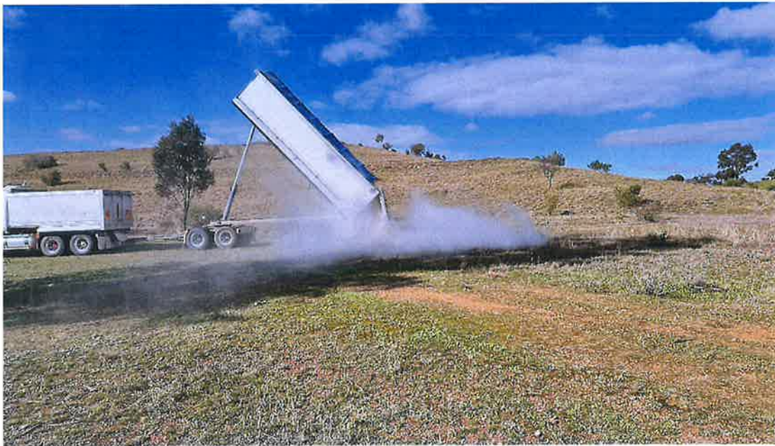
Photo 8: 105 tonnes of Ag lime from Parkes was delivered to site and spread on the heap leach and WRE in July 2025.
