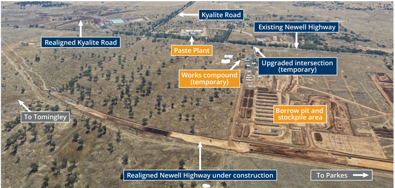
Construction zone: Tomingley Gold Extension Project
