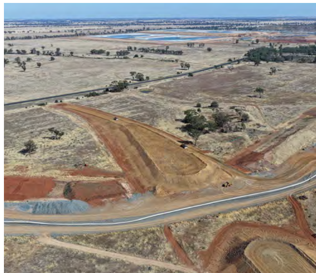
Northwest view of Kyalite Rd diversion, showing earthworks for the overpass.
