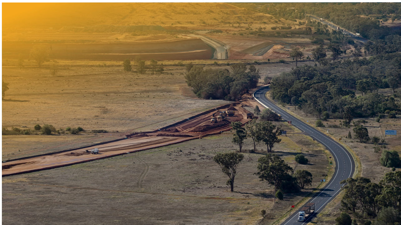
New section of Newell Highway under construction
