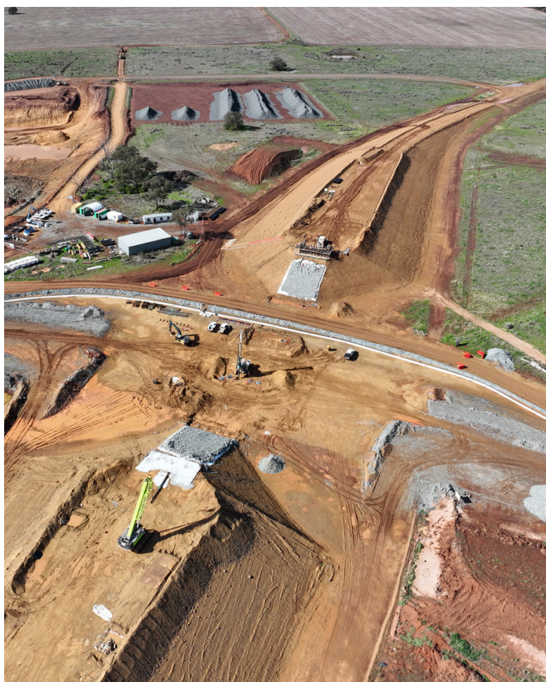
Kyalite Road overpass under construction
